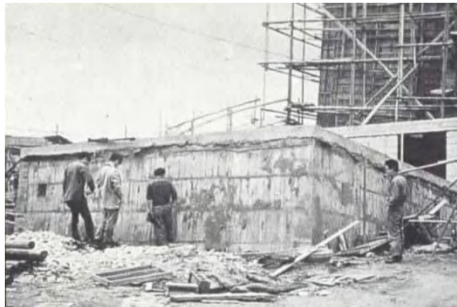
buried water tank floated up in Niigata Port, during 1964 Niigata Earthquake
