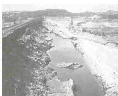
Slide in the Lower San Fernando Dam during 1971 San Francisco Earthquake
